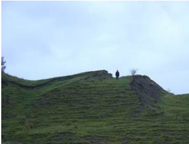
Photograph 3: Deep slide of the Mieg waste heap, Pechelbronn mining basin, Alsace (image: GEODERIS)
