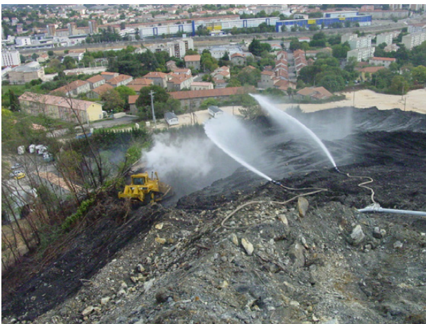
Photograph 5: Discharging and spraying a burning waste heap, Gard mining basin
