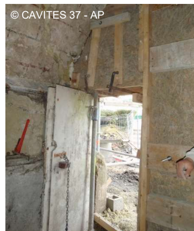
ROCHECORBON (37) – Appui coffré
