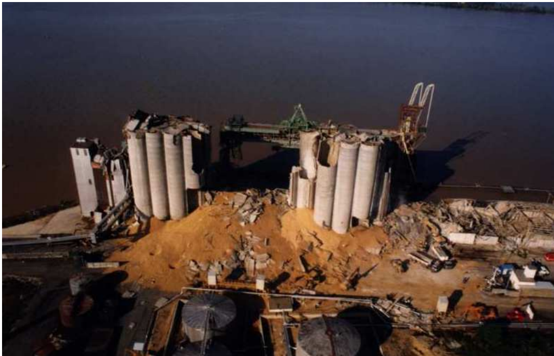
Figure 6: Silo at Blaye after the explosion of 20/08/1997 (excerpt from the detailed sheet ARIA of the BARPI downloadable at http://www.aria.developpement-durable.gouv.fr , accident n°11657)
