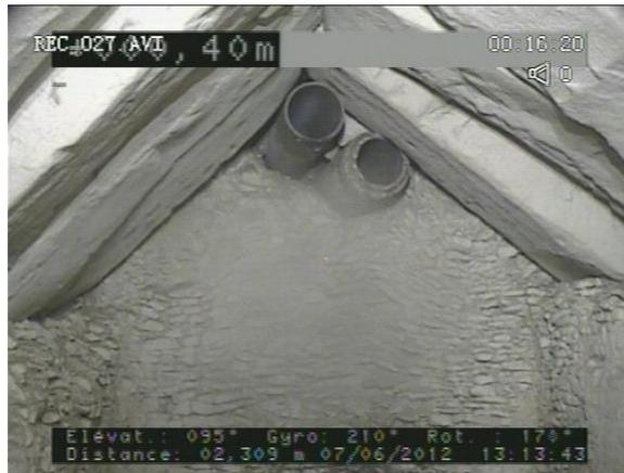
Digital picture taken by the acquisition card (example of closure of the head of an old shaft)
