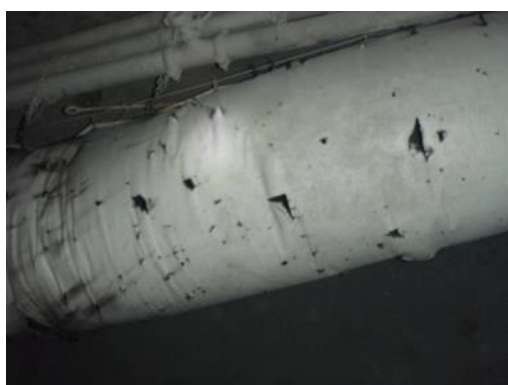
Figure 7. Exemples de gaines de ventilation souples percées (source : Auxiliary Ventilation: Good Installation and Maintenance Practices for Miners, Workplace Safety North, 2021)
