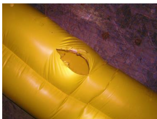
Figure 7. Exemples de gaines de ventilation souples percées (source : Auxiliary Ventilation: Good Installation and Maintenance Practices for Miners, Workplace Safety North, 2021)
