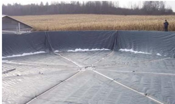
*Figure 10: Couverture souple flottante
