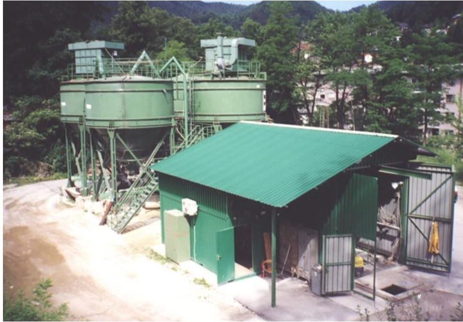
Fig. 6.4. Mixing plant, pumping station and control centre on surface (By courtesy of Bojan Rezùn).
