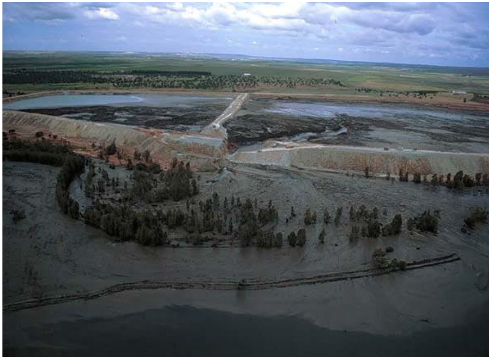
Figure 4.30. View of the Aznalcóllar dam failure consequences. (Source http://edafologia.ugr.es/donana/recursos/presa.jpg ).
