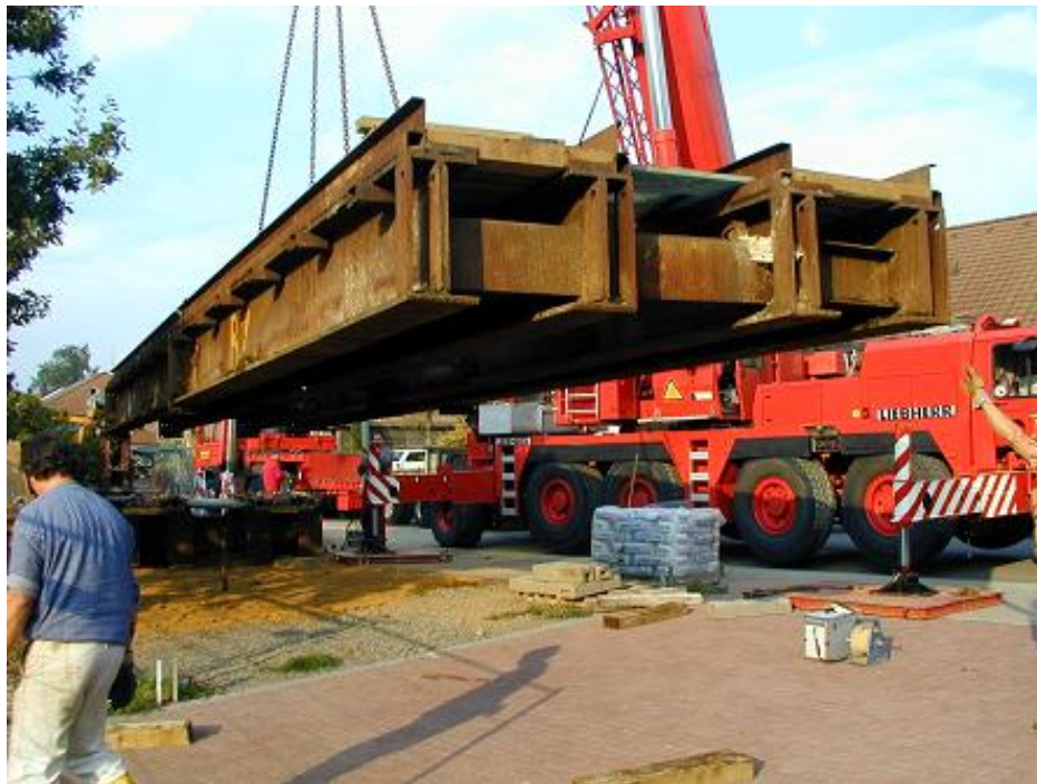
Figure 6.13. Steel platform positioned above a shaft (Source IHS, Aachen).
