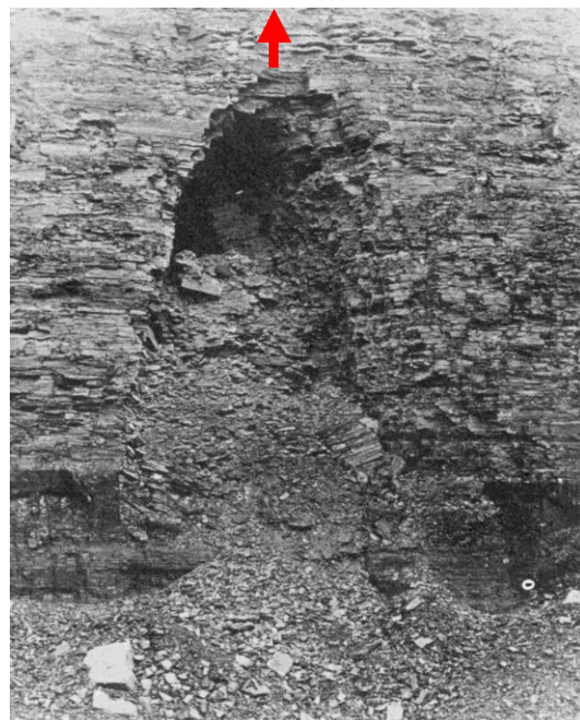
Figure 4.11. Examples of chimneying development in underground mining works
