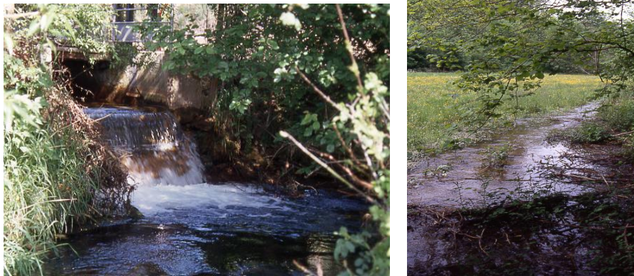
Figure 2.9. Discharge through an adit (left) and (right) development of a wet zone close to an other adit (Didier & Leloup, 2006)
