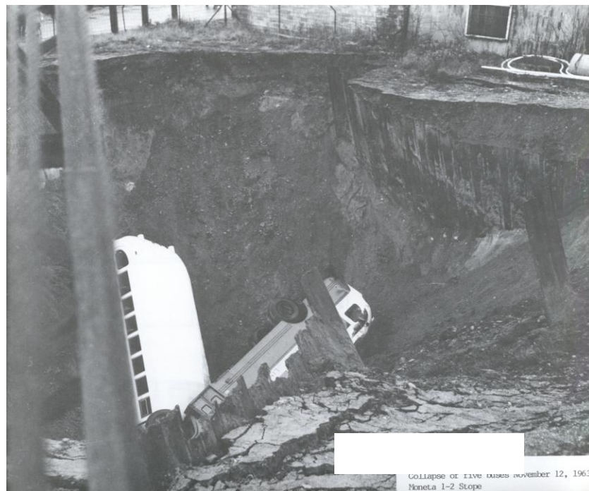
Figure 4.21. Consequence of sudden stope fill collapse, Moneta gold mine, Ontario (Hunt, 1989).
