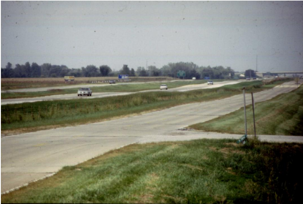
Figure 4.1. Example of subsidence effect on a motorway.
