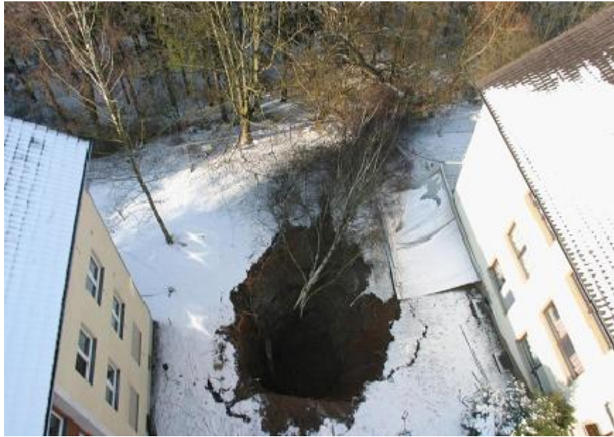
Figure 4.16. Sinkhole resulting of a shaft failure (Source BZR Arnsberg).
