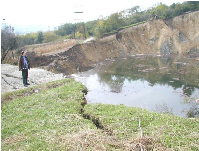
Figure 4.27. Collapse of the salt cavern of Ocnele Mari – Romania (By courtesy of Bernard Feuga).
