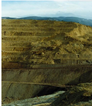
Figure 4.29. Slope failure in a French open pit mine (Source CdF).
