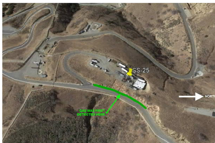
Figure 2: Location of the first gas leak zone on 23 October 2015 [14]
